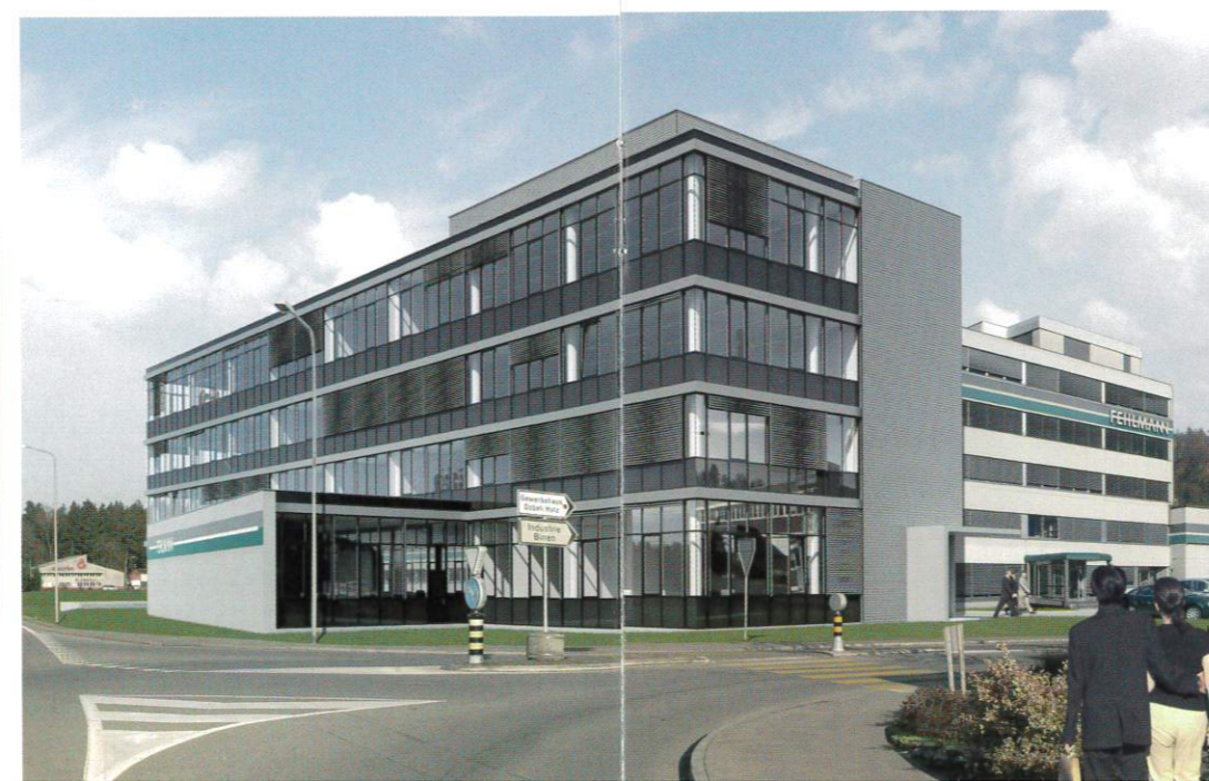
The just finished Fehlmann Technology Center setting new standards throughout
